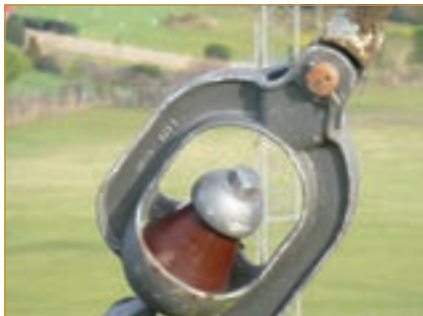
Imagery from a Sky-Futures UAS is able to provide sufficient detail to show the identification numbers on a cable. (Photo: Sky-Futures)
